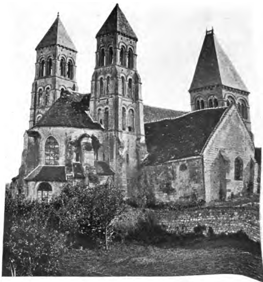
MORIENVAL ABBEY CHURCH (c. 1125) BEFORE "RESTORATION"
